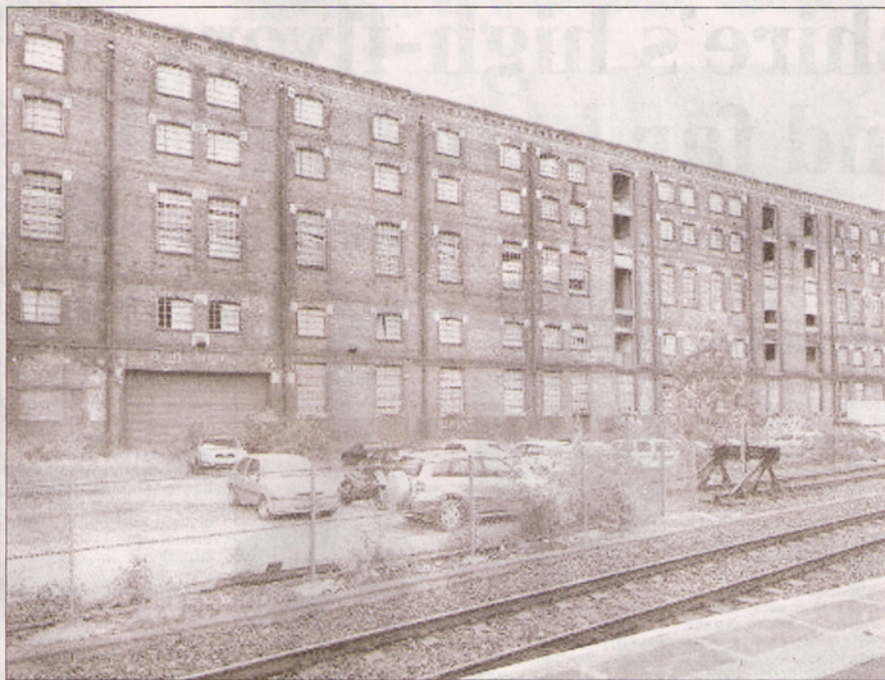
St George's Warehouse, in Huddersfield.
